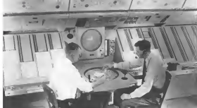
Continues one traffic display scope for plotting and scope are wall for use all view in Raytheon-developed system now installed at Indianapolis' new Air Route Traffic Control Center. This is the first of 60 bright display systems developed for FAA.
